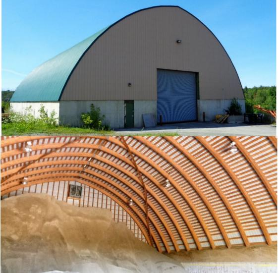
**Definition:** Building is framed with heavy timbers, laminated veneer lumber (LVL), or steel. The internal frame work supports the building, and is sheathed with steel panels or plywood and asphalt shingles.
