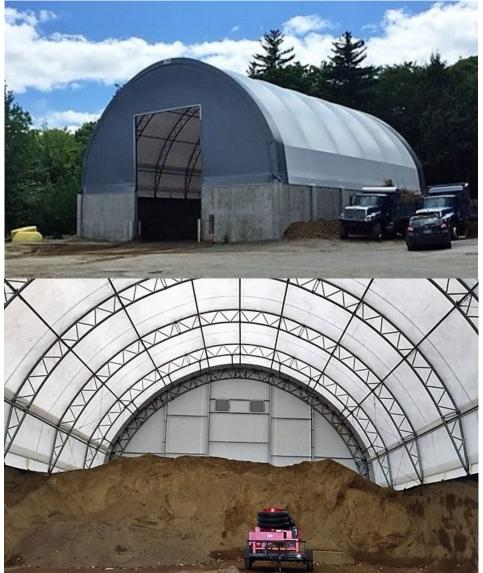
**Definition:** Building is framed with aluminum tubing on a poured formed concrete foundation. The internal frame work supports the building. The exterior is sheathed with fabric stretched taut with ratchet straps located along the foundation perimeter.
