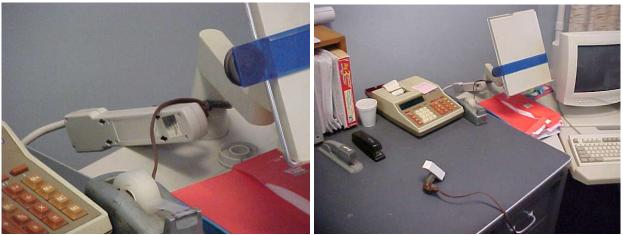
A potential tragedy in a Maine town office. A multiple outlet strip with a "zip cord" extension cord, ground "cheater", and triple outlet adaptor. Depending on the appliances plugged into this setup, it could pose both a serious fire and electrocution hazard!
