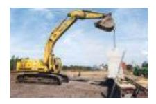
It may be a load under a mobile crane, an overhead hoist in the shop, or a culvert or trench box under a loader bucket, but anytime there is a load in the air, there is a very serious hazard. Everyone, including the equipment operator, rigger, and other workers in the area must pay special attention if everyone is going to go home at the end of the shift!
